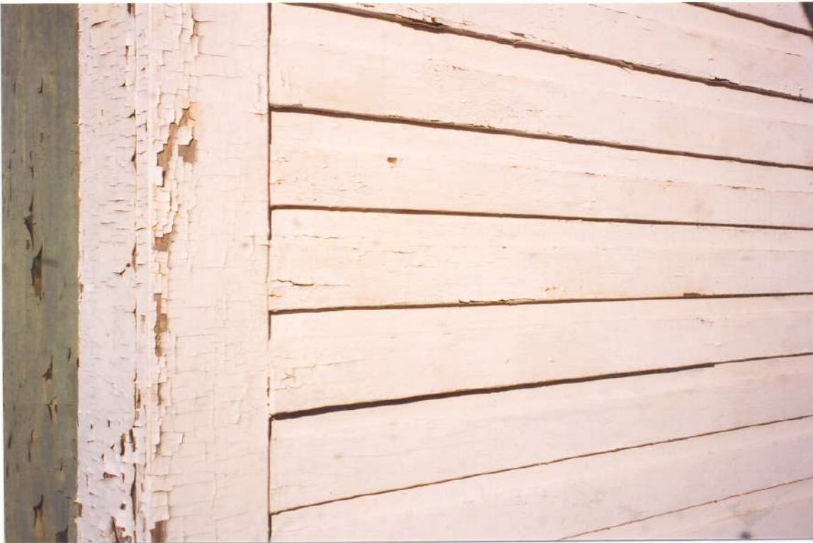
Figure 80. Garage: North elevation, detail of novelty siding (1999).
