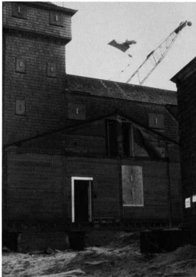
Illustration 27. Separation of Boat Room from Main Structure, November 1977.
