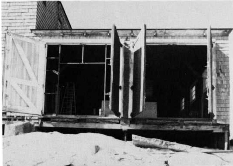
Illustration 26. North-Elevation Boat Room Doorways, Framing for Screen Within Doorway 115.
