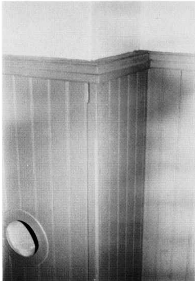
Illustration 38. Mess Room: Reproduction Chimney Wainscot With Original Corner Piece.
