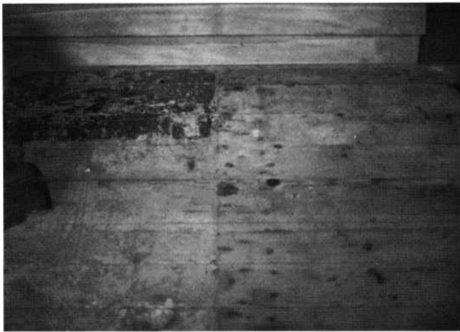
Illustration 24. Boat Room Floor, Looking East at Paint Evidence of Storeroom in Southeast Corner.
