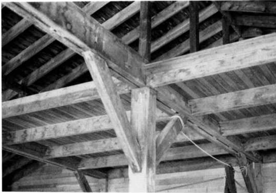
Illustration 48. Boat Room: Roof Truss and Post.
