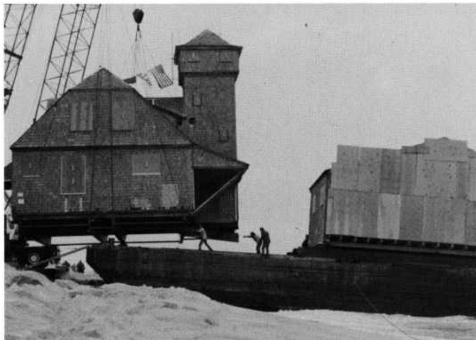
Illustration 28. Loading Boat Room and Main Structure onto Barge, November 30, 1977.
