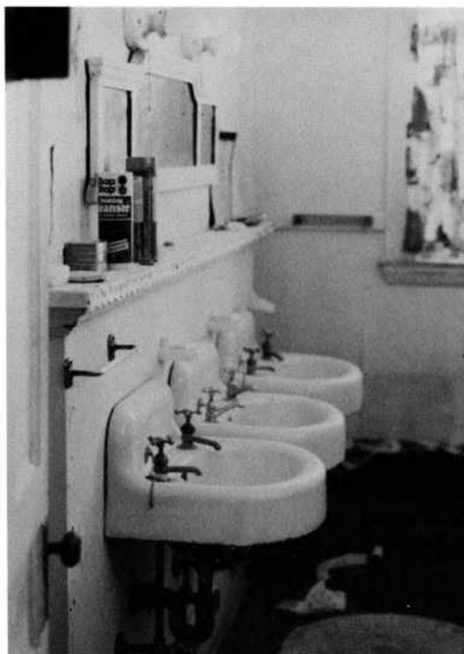
Illustration 18. East Wall of Spare Room, Sinks Installed During 1942 Improvement to Second-Floor Bathroom.
