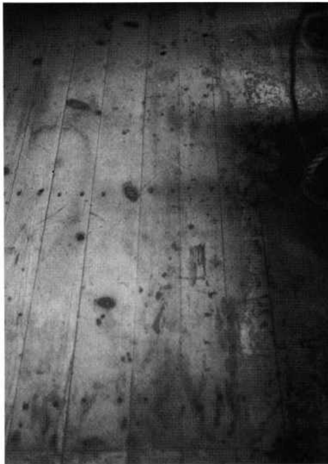
Illustration 25. Boat Room Floor, Looking South at Paint Evidence of Storeroom in Southeast Corner.
