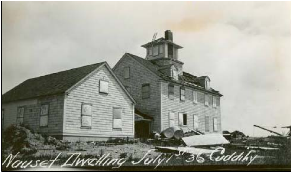
Figure 2.23. Nauset Coast Guard Station, construction, July 1, 1936.
