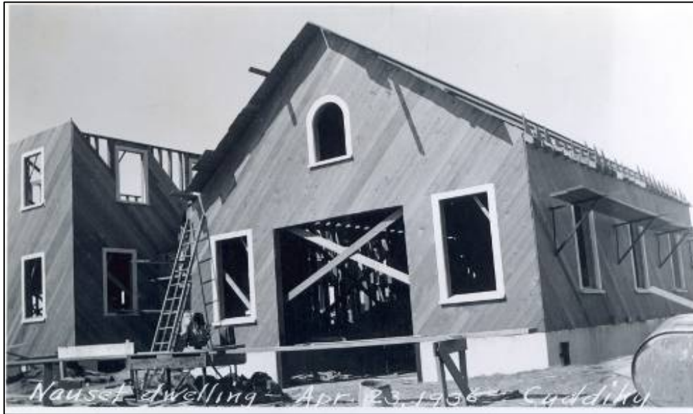
Figure 2.07. Nauset Coast Guard Station, balloon- frame construction, northeast corner of boathouse, April 23, 1936.
