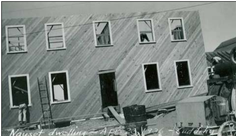
Figure 2.06. Nauset Coast Guard Station, balloon- frame construction, south façade, April 23, 1936.
