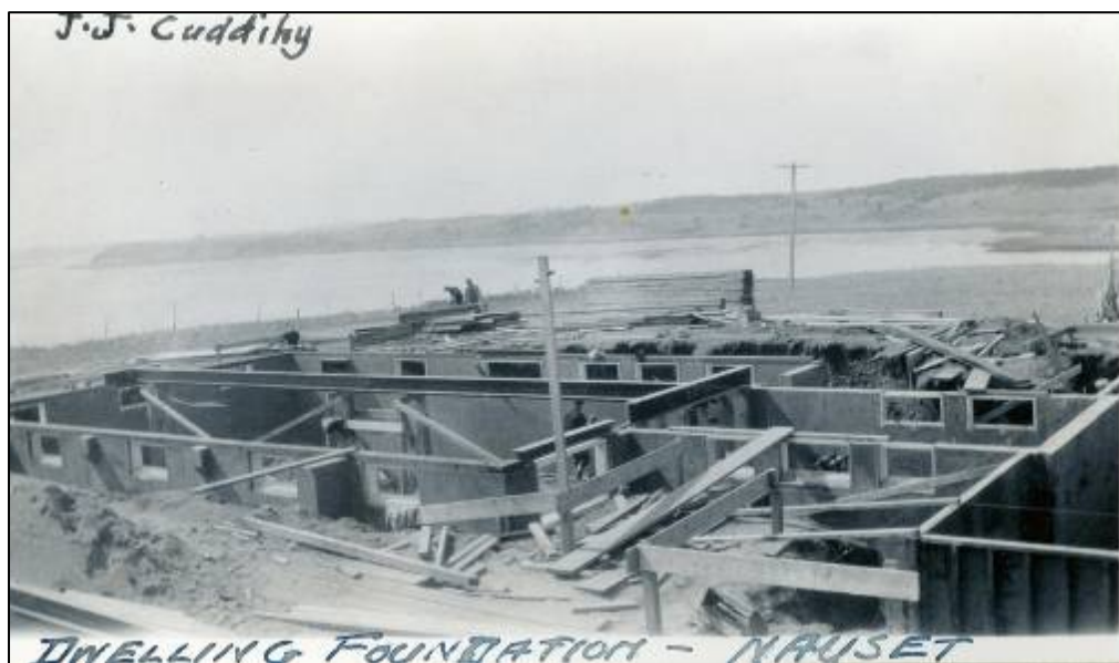
Figure 2.04. Nauset Coast Guard Station, foundation construction looking southwest, circa March or April 1936.
