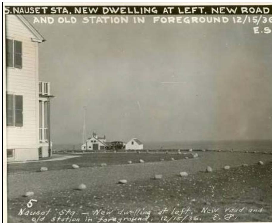
Figure 2.33. Nauset Station, new dwelling and new road after completion, December 15, 1936. The old station is seen in the background.
