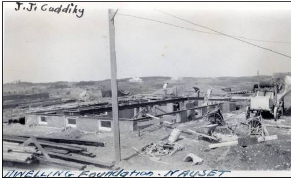
Figure 2.03. Nauset Coast Guard Station, foundation construction looking northwest, circa March or April 1936.
