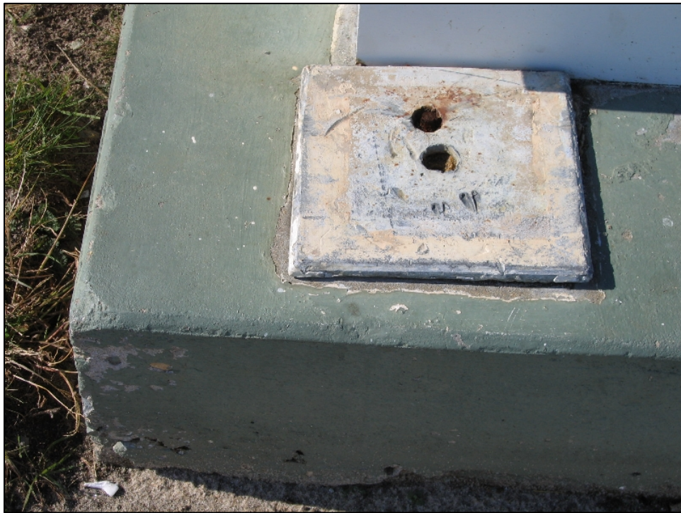
Figure 4.22. Front porch, typical slate base for handrail newel post.
