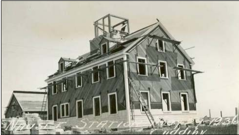
Figure 2.19. Nauset Coast Guard Station, construction, May 29, 1936.
