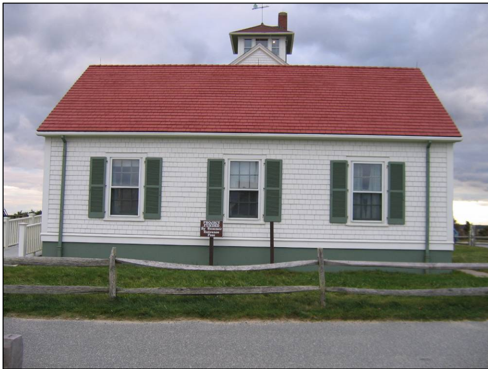
Figure 4.04. Boathouse, north elevation.
