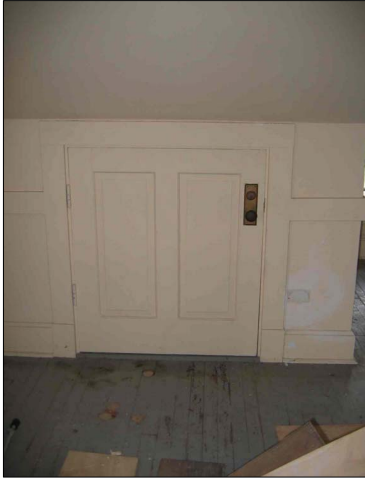
Figure 4.118. Room 303 (north loft room), doorway #3H.
