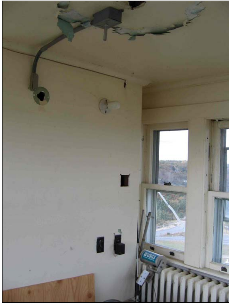
Figure 4.122. Room 401 (watch room), northwest corner.
