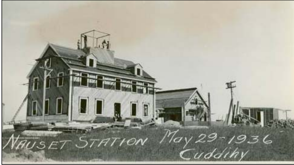
Figure 2.17. Nauset Coast Guard Station, construction, May 29, 1936.
