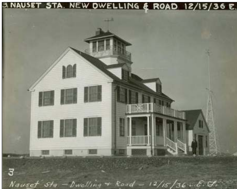
Figure 2.31. Nauset Station, new dwelling and road after completion, December 15, 1936.
