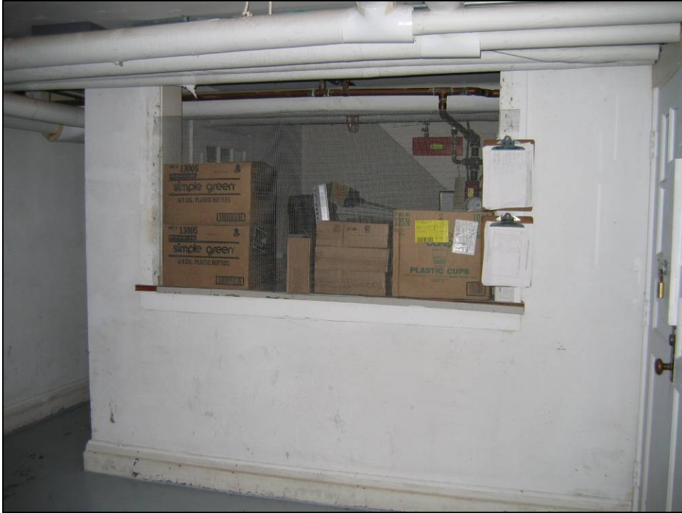
Figure 4.43. Room 08 (shop and drill room), west wall, borrowed- light window.
