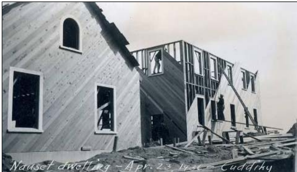
Figure 2.08. Nauset Coast Guard Station, balloon- frame construction, north elevation viewed from the northwest, April 23, 1936.
