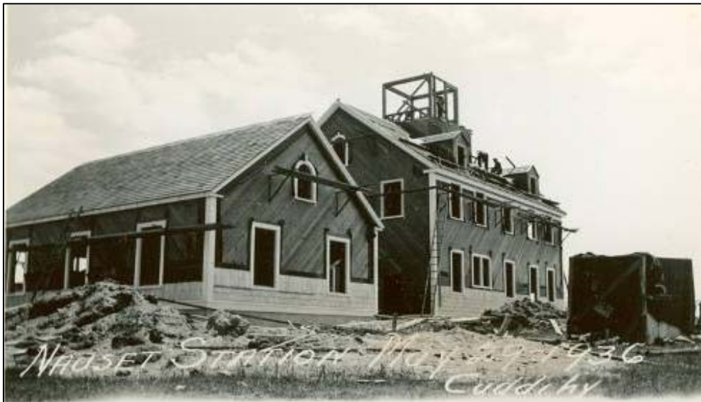
Figure 2.20. Nauset Coast Guard Station, construction, May 29, 1936.
