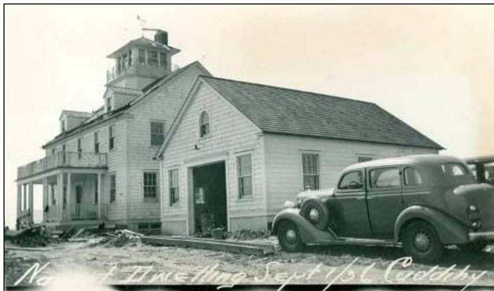
Figure 2.26. Nauset Coast Guard Station, construction, September 1, 1936.
