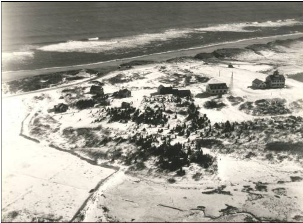
Figure 2.50. Nauset Coast Guard Station, aerial view from the northwest, circa 1961.
