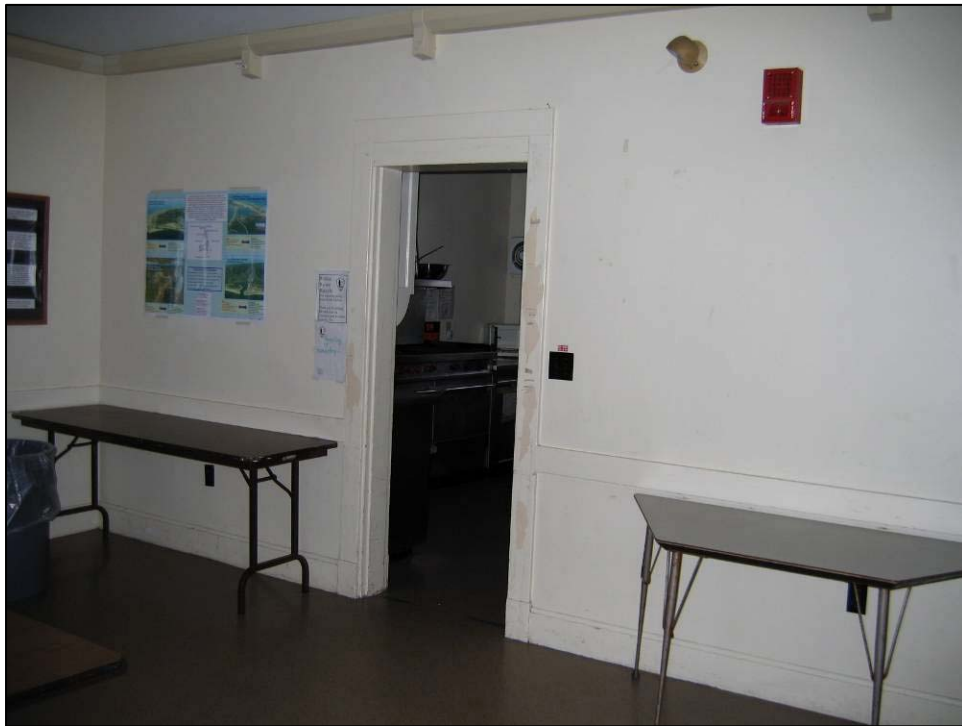
Figure 4.59. Room 102 (mess room), west wall and doorway #1J.
