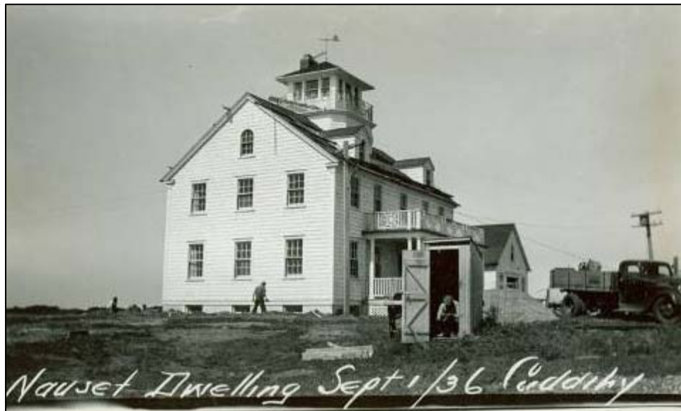
Figure 2.25. Nauset Coast Guard Station, construction, September 1, 1936.
