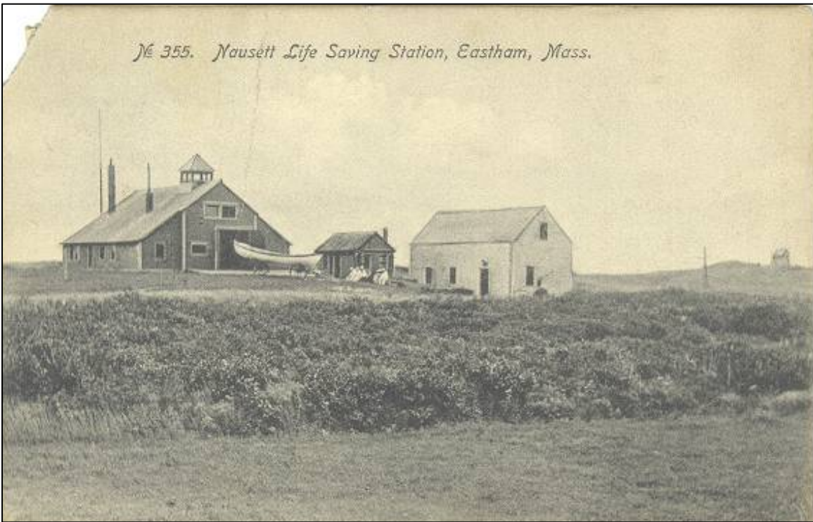
Figure 1.03. Expanded Red House- type Lifesaving Station at Nauset, view from the northwest, circa 1887- 1907.
