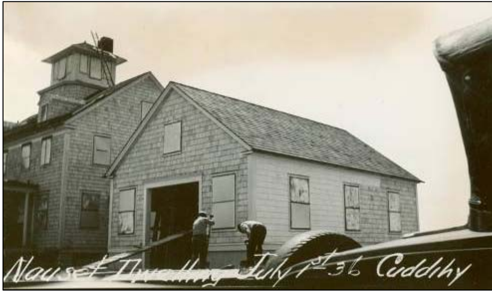
Figure 2.21. Nauset Coast Guard Station, construction, July 1, 1936.
