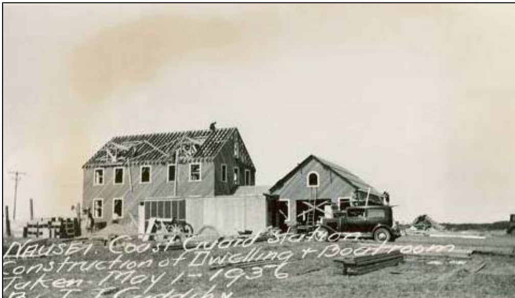
Figure 2.12. Nauset Coast Guard Station, construction, May 1, 1936.
