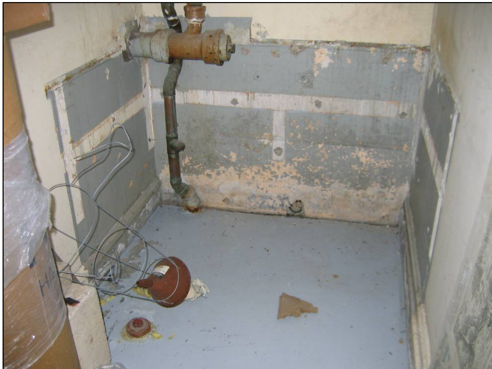
Figure 4.46. Room 010 (provisions room), west wall.
