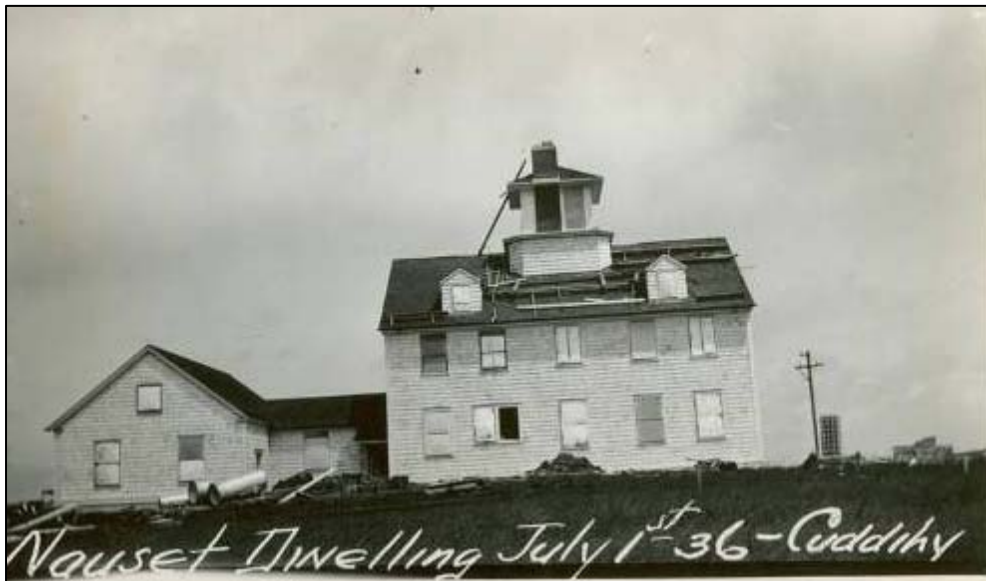
Figure 2.24. Nauset Coast Guard Station, construction, July 1, 1936.
