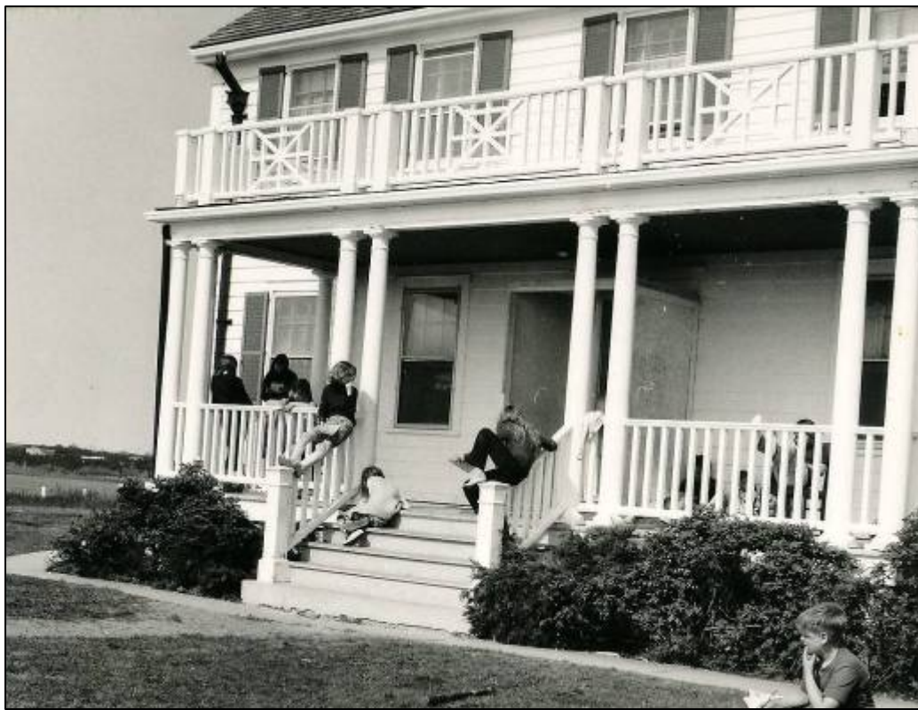
Figure 2.54. Nauset Coast Guard Station, front porch, circa 1970- 71.
