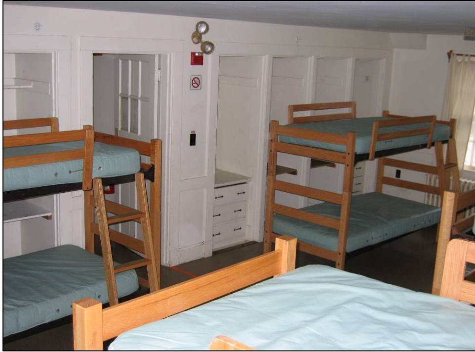
Figure 4.91. Room 202 (dormitory), south wall, southwest corner.
