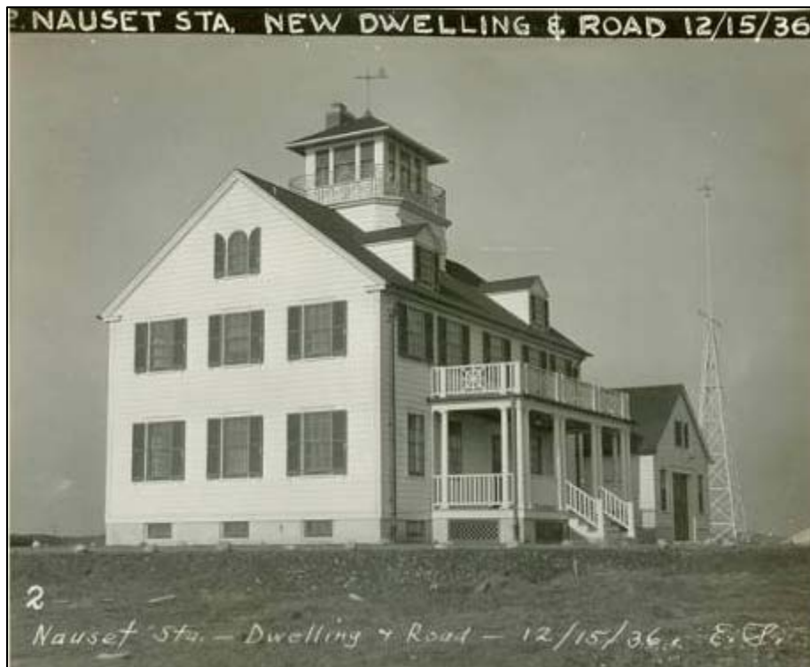
Figure 2.30. Nauset Station, new dwelling and road after completion, December 15, 1936.
