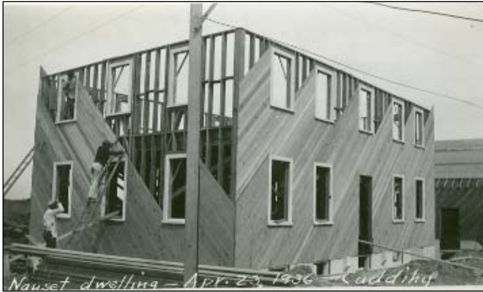
Figure 2.05. Nauset Coast Guard Station, balloon- frame construction, southeast corner of dwelling, April 23, 1936.
