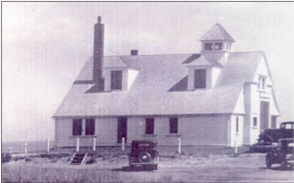
Figure 1.09. Expanded Red House- type Lifesaving Station at Nauset, view from the northwest, circa 1930.
