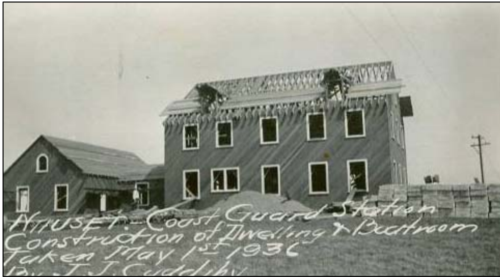
Figure 2.13. Nauset Coast Guard Station, construction, May 1, 1936.
