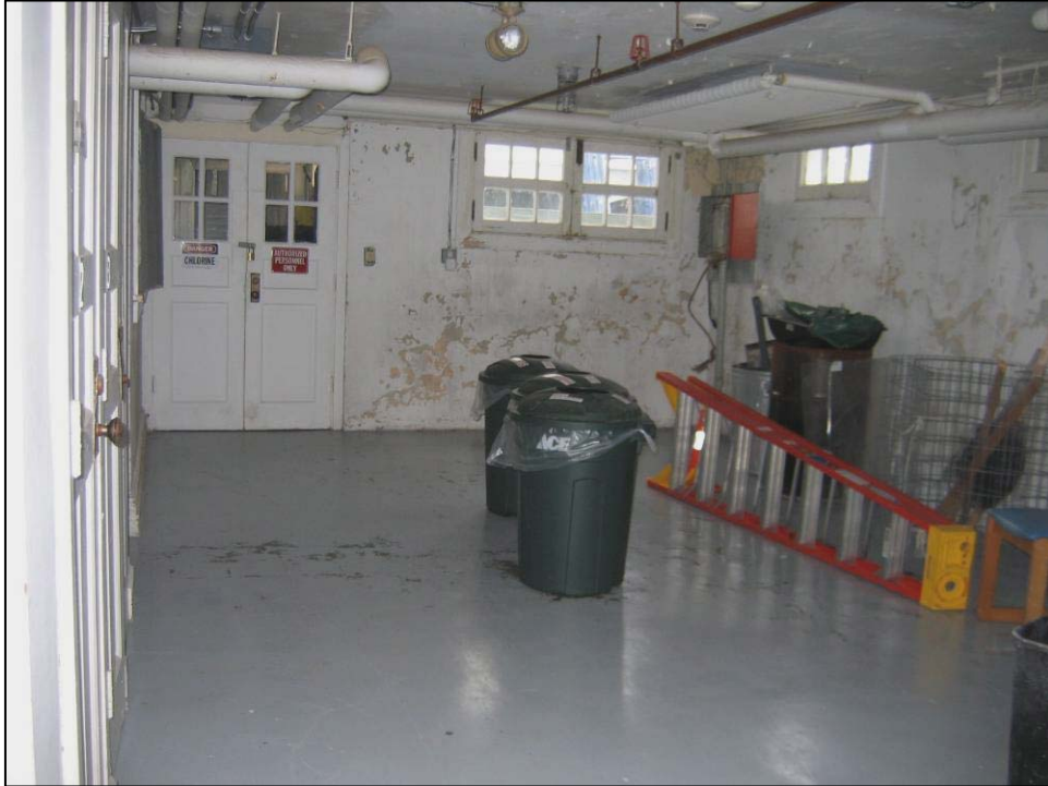
Figure 4.45. Room 08 (shop and drill room), northeast corner.
