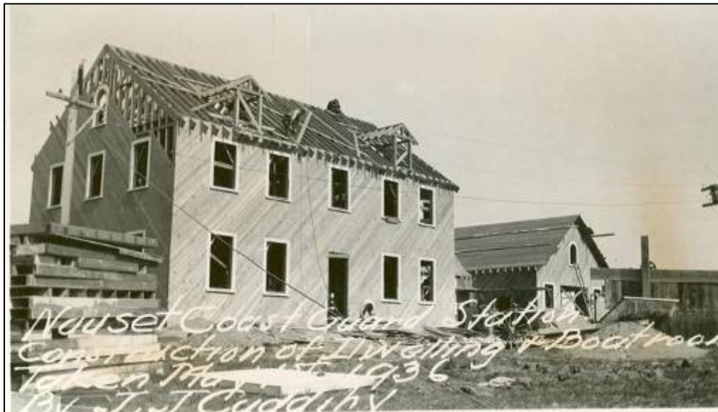
Figure 2.10. Nauset Coast Guard Station, construction, May 1, 1936.
