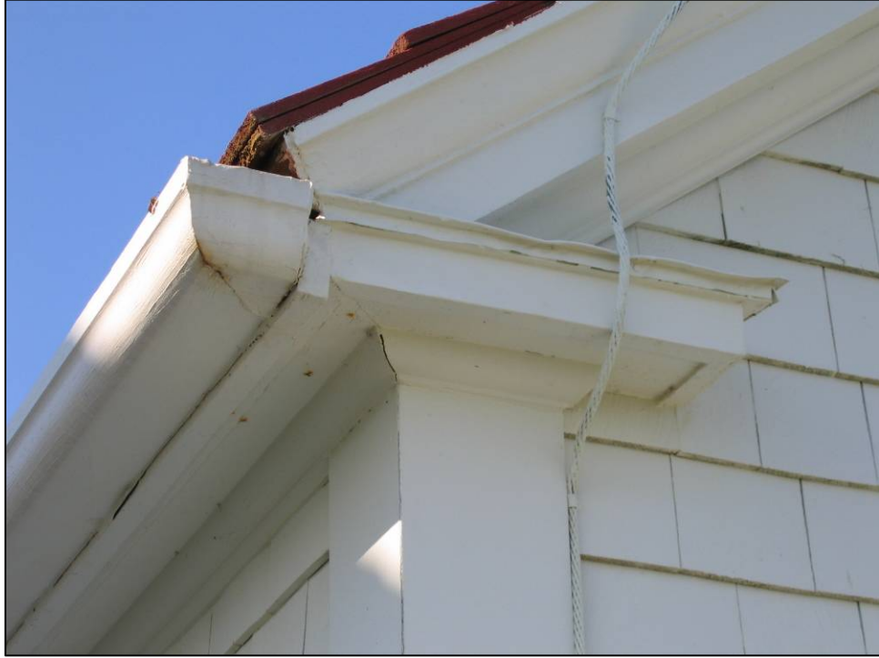
Figure 4.09. Dwelling, eave at southwest corner.
