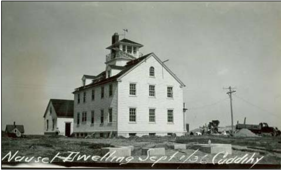
Figure 2.27. Nauset Coast Guard Station, construction, September 1, 1936.
