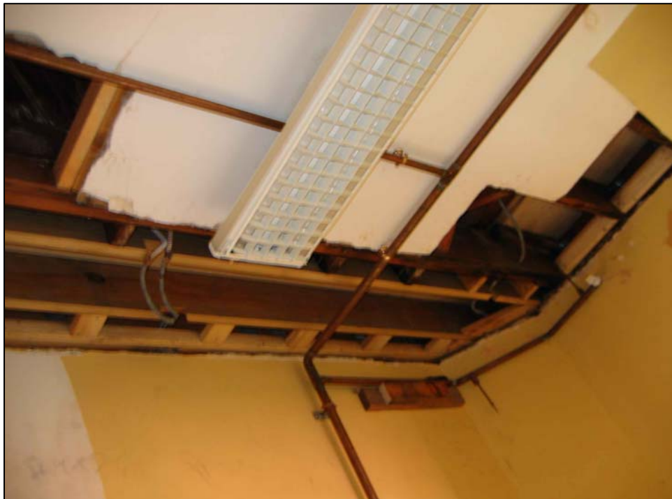
Figure 4.113. Room 301 (loft stair hall), ceiling damage at southwest corner.
