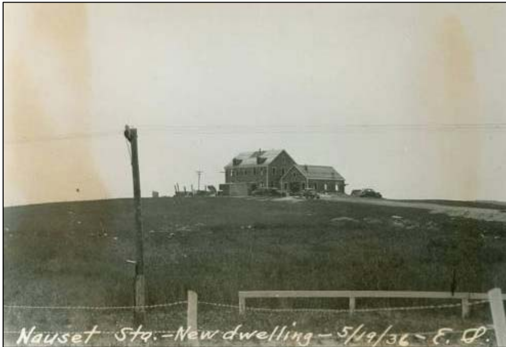
Figure 2.15. Nauset Coast Guard Station, construction, May 19, 1936.
