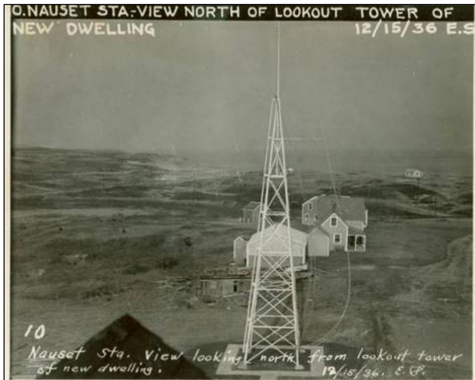
Figure 2.37. Nauset Station, view north from lookout tower of new dwelling, December 15, 1936.
