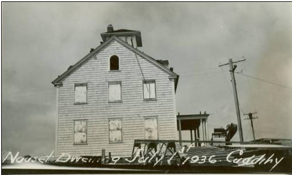
Figure 2.22. Nauset Coast Guard Station, construction, July 1, 1936.
