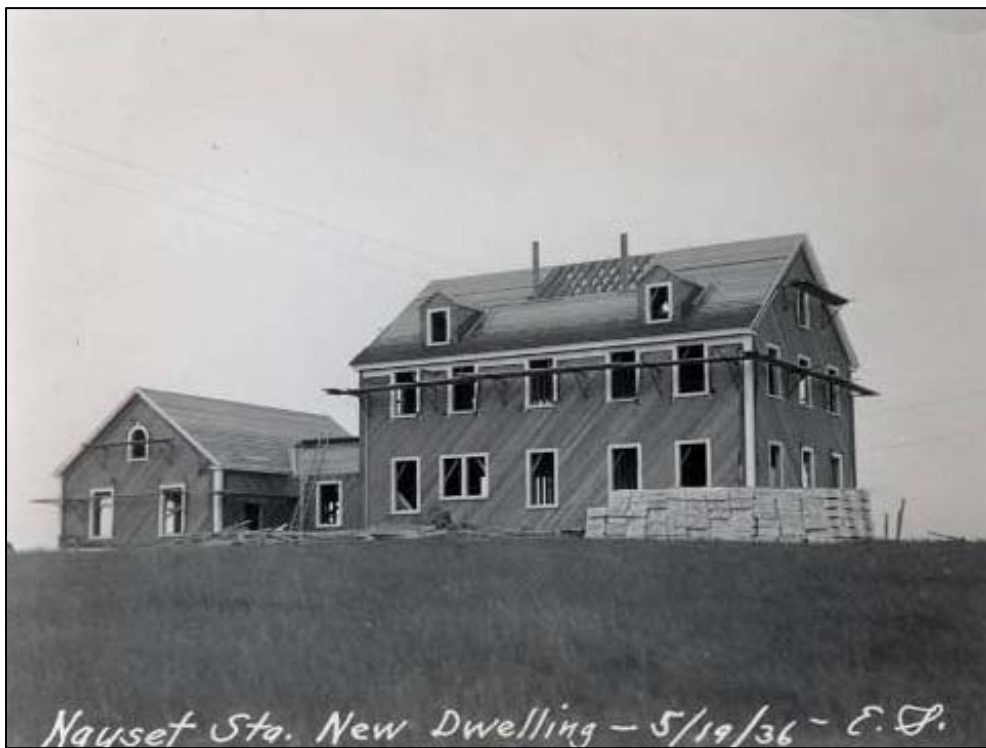
Figure 2.16. Nauset Coast Guard Station, construction, May 19, 1936.
