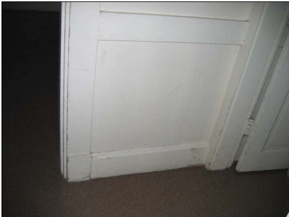
Figure 4.71. Room 107 (passageway), north wall, northeast corner.
