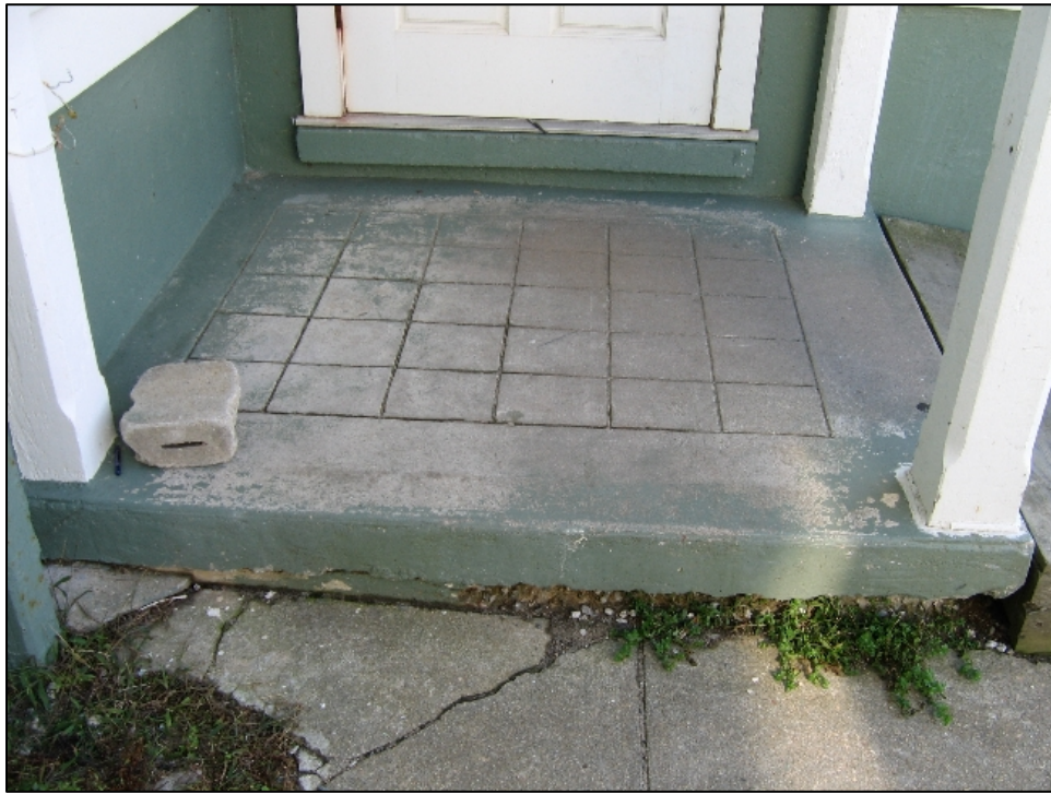
Figure 4.21. Kitchen entry porch, scored concrete slab.
