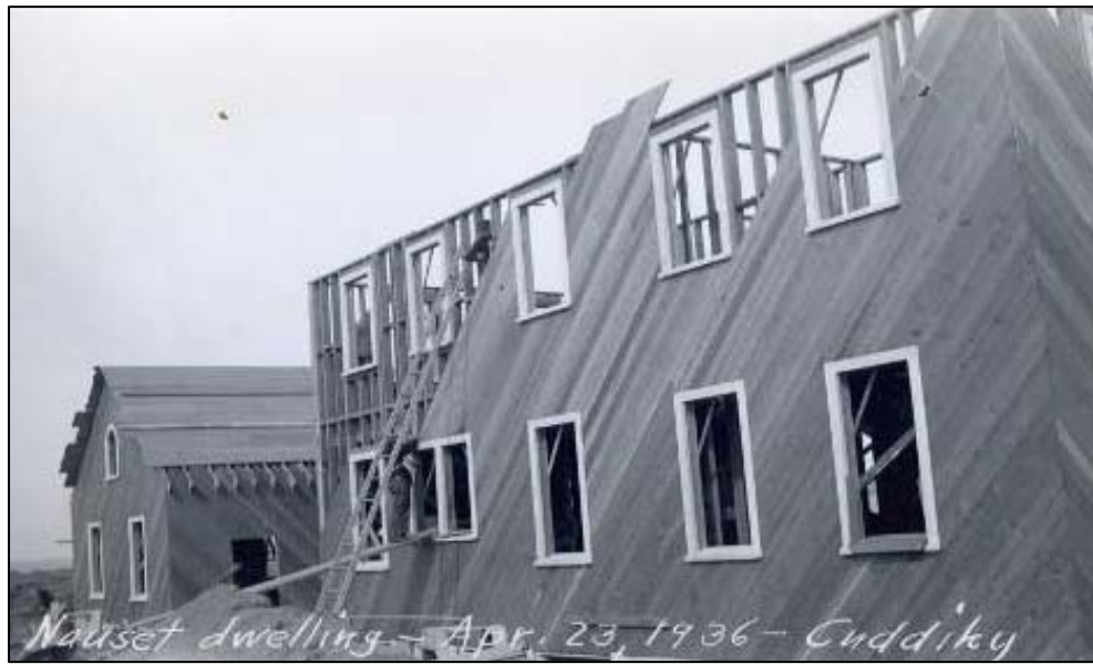
Figure 2.09. Nauset Coast Guard Station, balloon- frame construction, north elevation viewed from the southwest, April 23, 1936.
