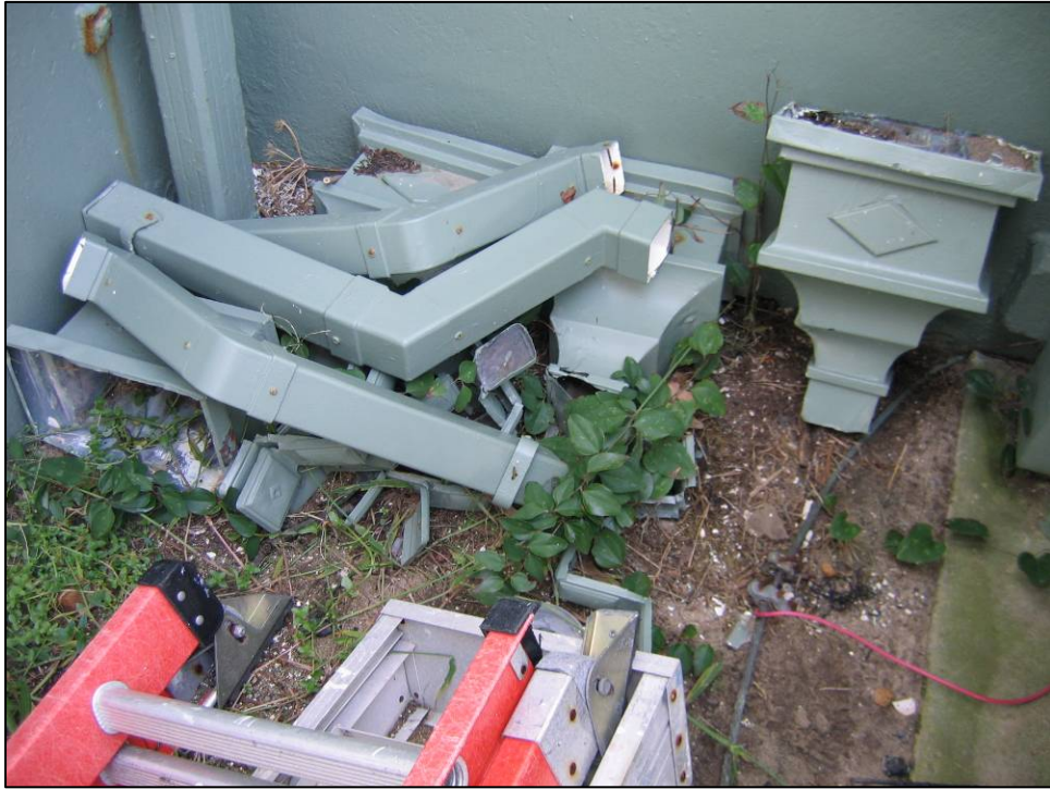
Figure 4.10. Stockpiled roof drainage accessories.
