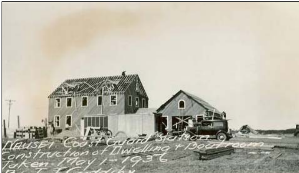
Figure 2.14. Nauset Coast Guard Station, construction, May 1, 1936.
