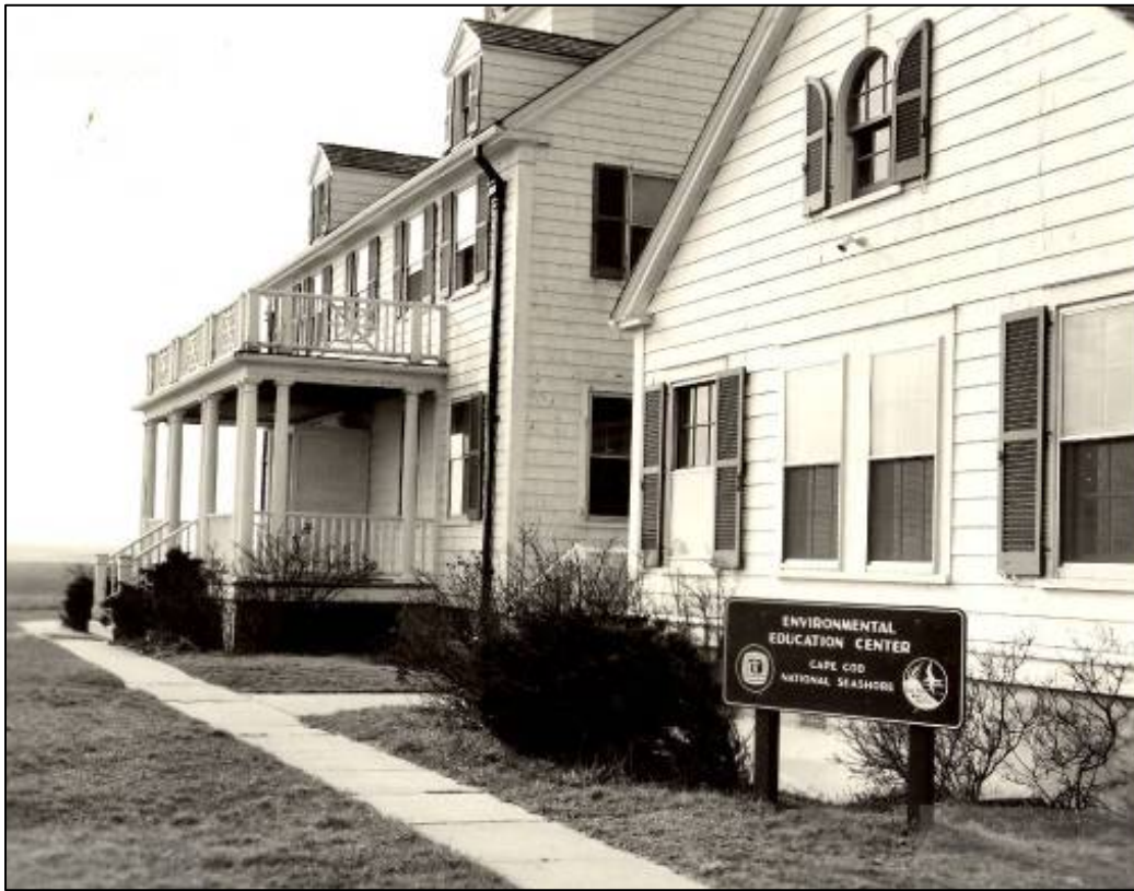
Figure 2.57. Nauset Coast Guard Station, east elevation, 1972.
