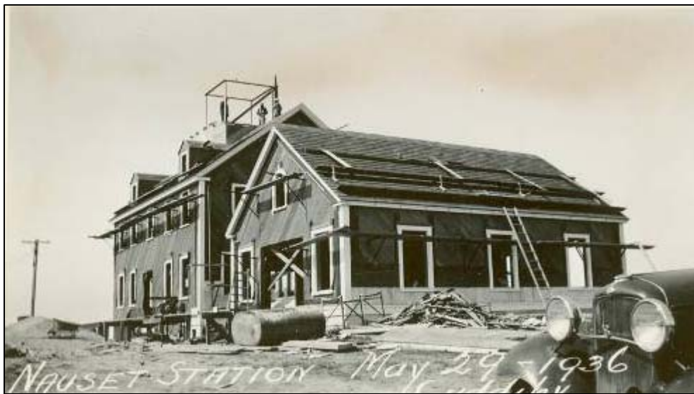
Figure 2.18. Nauset Coast Guard Station, construction, May 29, 1936.
