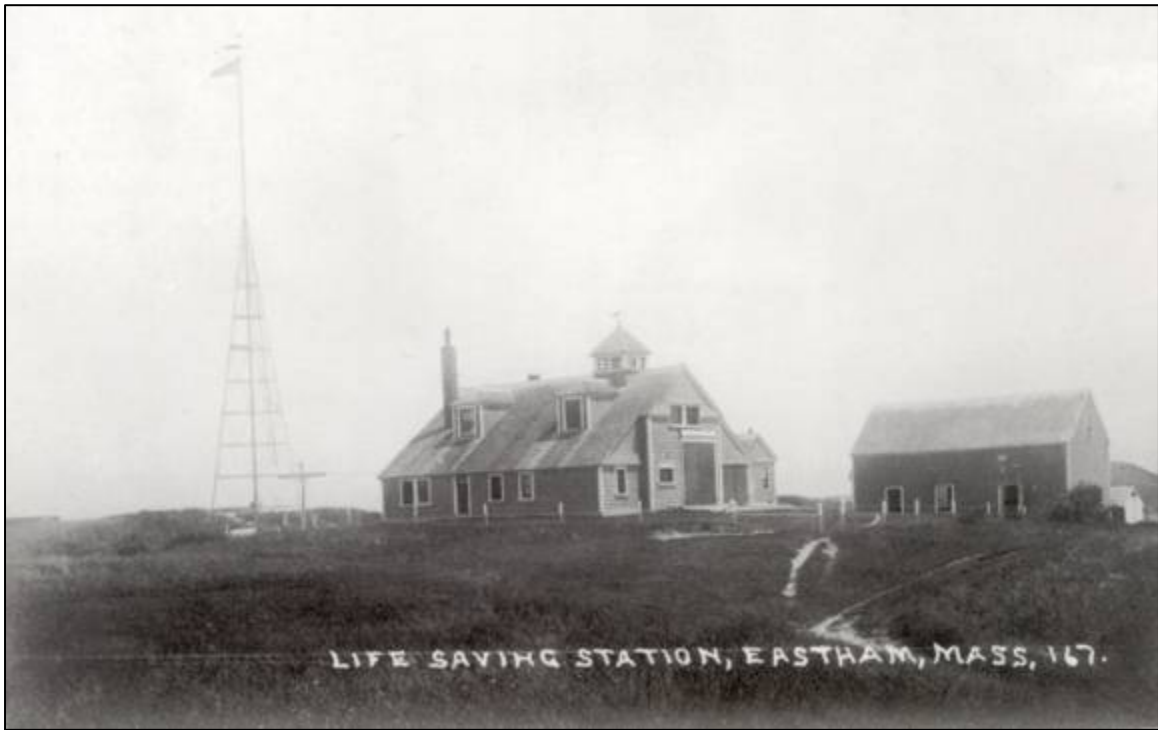
Figure 1.08. Expanded Red House- type Lifesaving Station at Nauset, view from the northwest, showing additional alterations after 1907.
