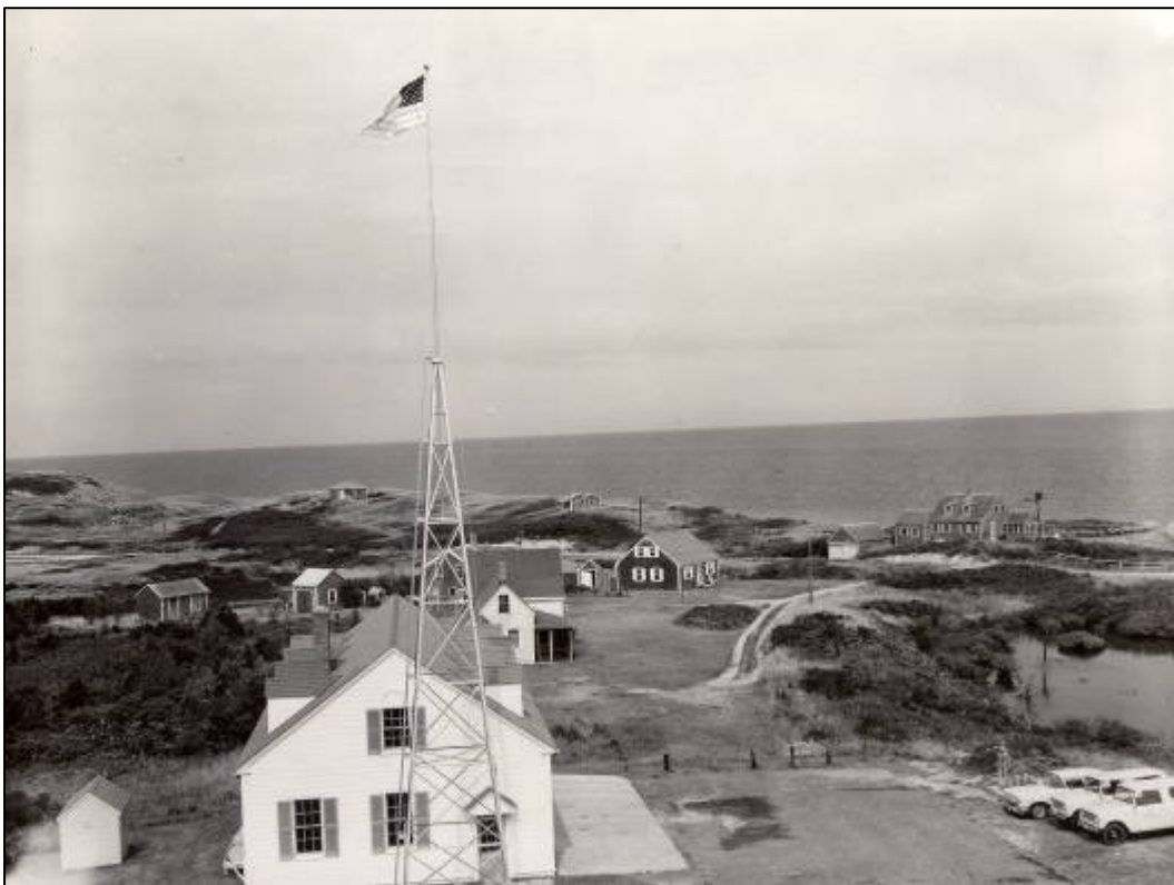
Figure 2.51. Nauset Coast Guard Station, view northward from the watch room, circa 1960s.
