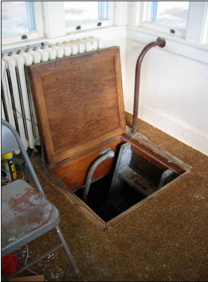
Figure 4.120. Room 401 (watch room), scuttle at northeast corner.
