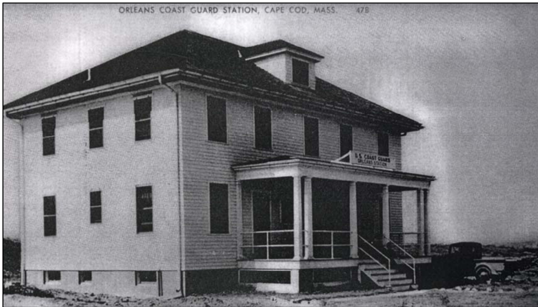
Figure 1.15. Modified Chatham- type Coast Guard Station: the “American Foursquare” variant at Orleans, MA, circa 1933.
