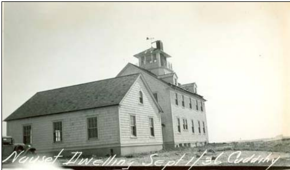
Figure 2.28. Nauset Coast Guard Station, construction, September 1, 1936.
