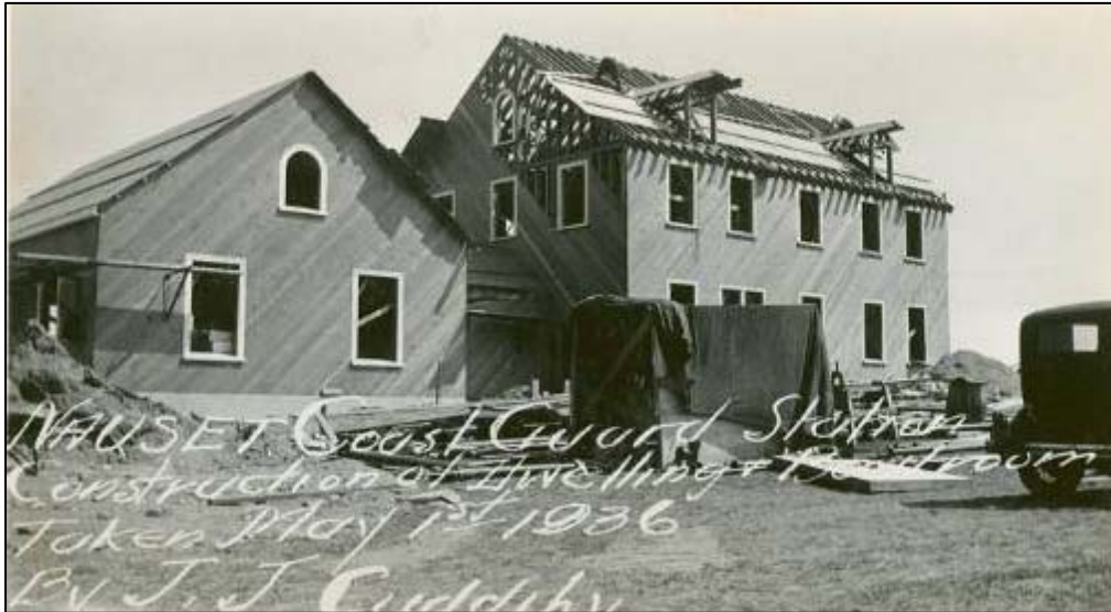
Figure 2.11. Nauset Coast Guard Station, construction, May 1, 1936.
