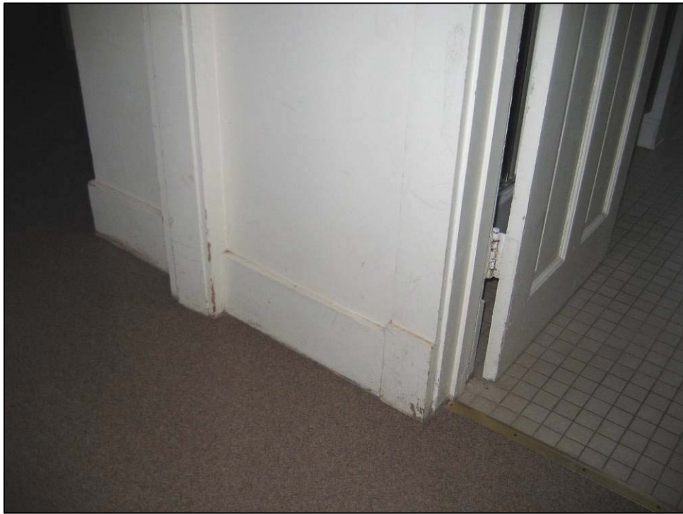
Figure 4.70. Room 107 (passageway), south wall, southeast corner.
