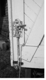
**FIGURE 81.** View of typical upper (left) and lower (right) sliding bolts on boat room doors. (T. Jones, NPS, 2005)
