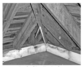
FIGURE 65. View of roof hip and junction of rafters and top plate of second floor walls. (T. Jones, NPS, 2005)
