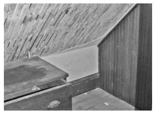
FIGURE 88. View of original plaster on wood lath in one of the closets in Room 201. (T. Jones, NPS, 2005)
