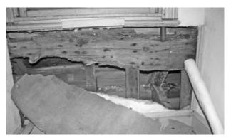
FIGURE 142. View damaged wall below window in Room 202. (T. Jones, NPS, 2005)
