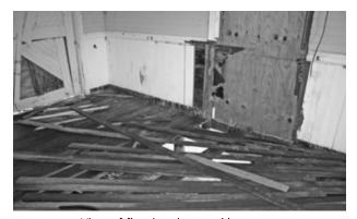
**FIGURE 121.** View of flooring damaged by storm surge in 1993. (T. Jones, NPS, 2005)
