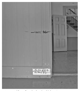
FIGURE 103. View of marks showing high-water marks for recent hurricanes. (T. Jones, NPS, 2005)
