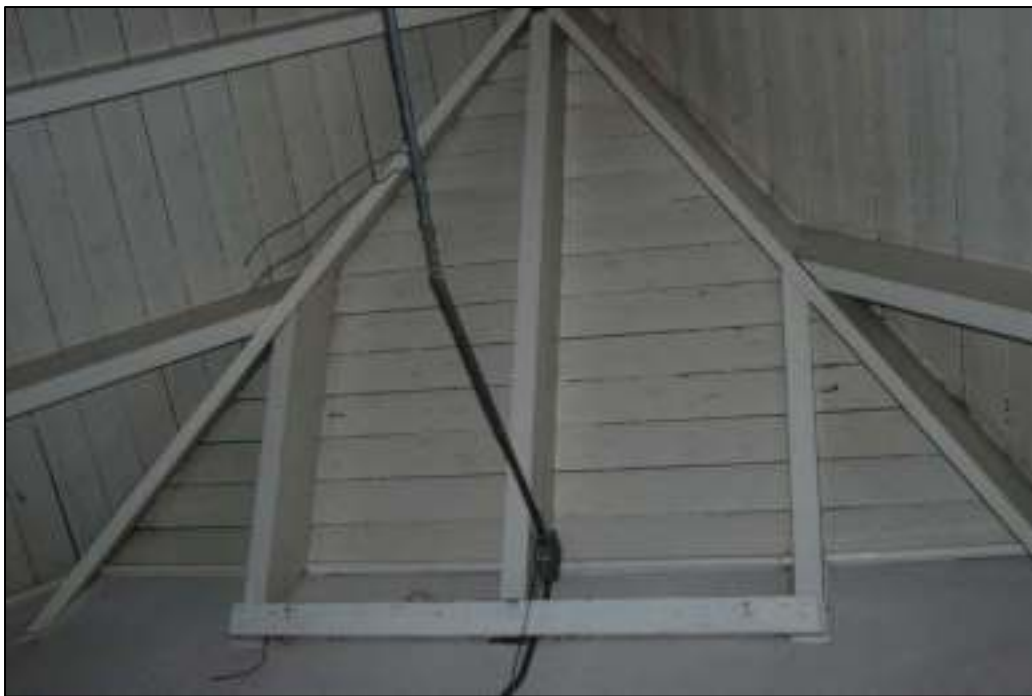
Figure 60. Spermaceti Cove Life-Saving Station, Room 206 interior view of clipped-gable roof framing looking south.
