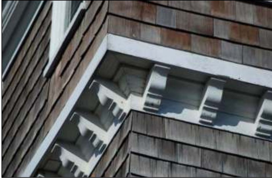
Figure 45. Spermaceti Cove Life-Saving Station, cornice below cantilevered section of Tower depicting brackets and molding.
