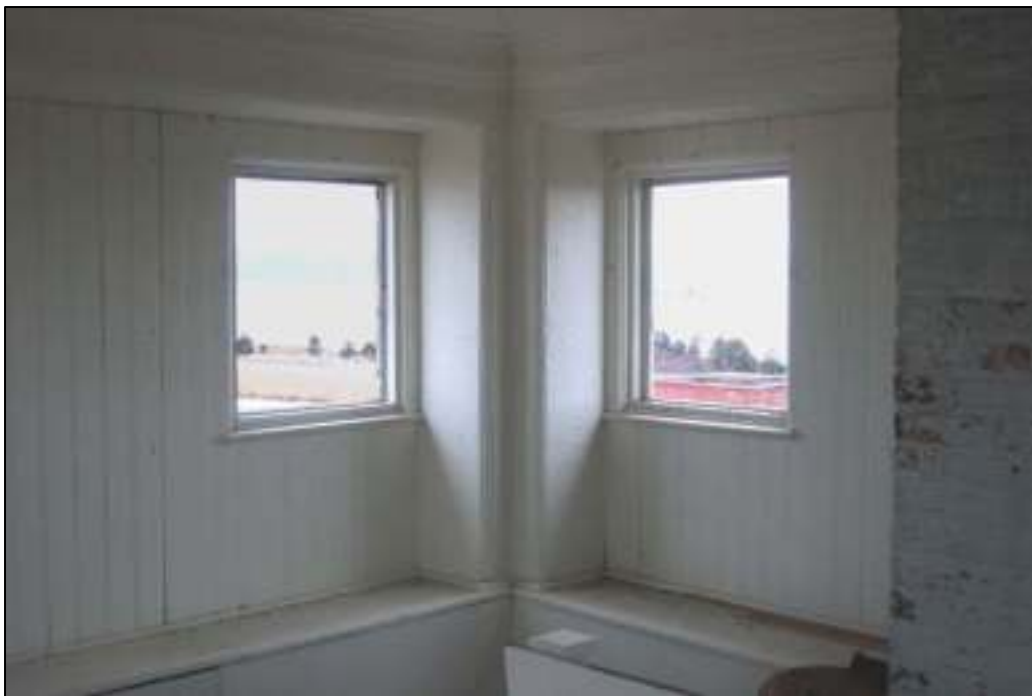
Figure 64. Spermaceti Cove Life-Saving Station, Watch Room/Room 401 looking southwest depicting cantilevered window section and typical woodwork for the fourth story.
